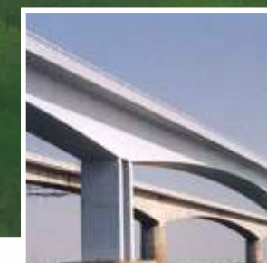
NAIGAON E/W BRIDGE
