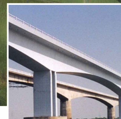
NAIGAON E/W BRIDGE
